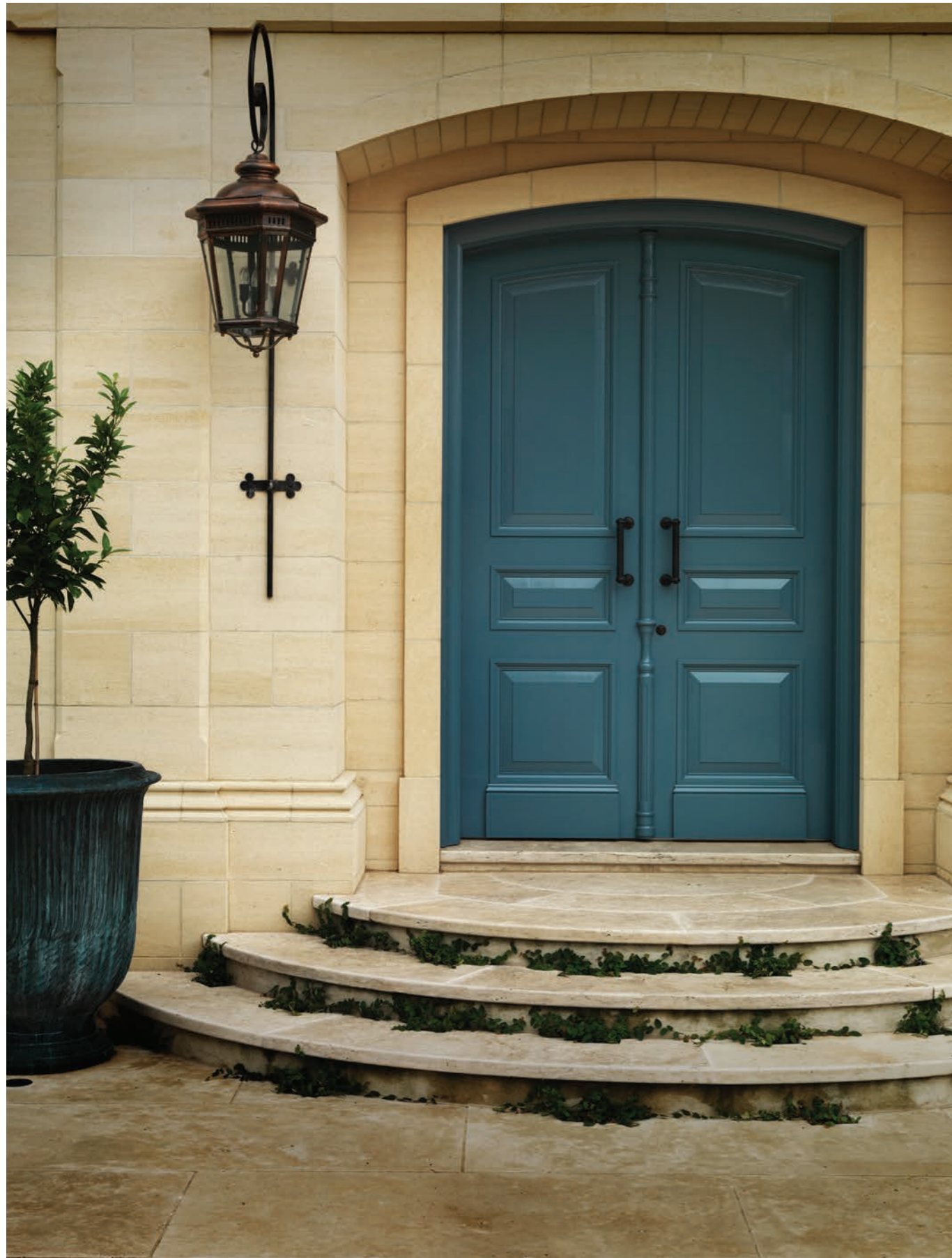
TUMBLLED WALNUT TRAVERTINE PAVING AND STEPS
