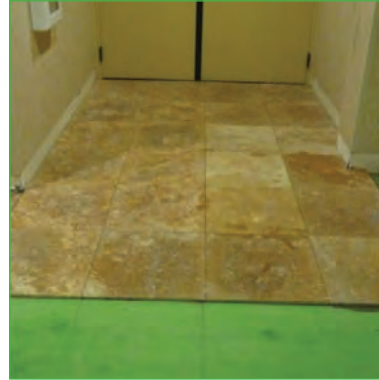
Lay Thinset and Flooring Directly on GreenSkin™
