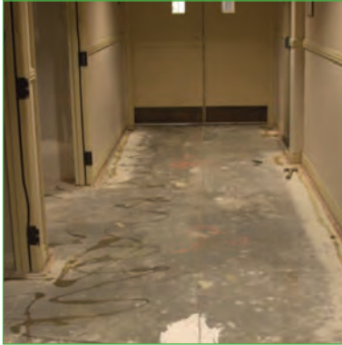
Wet Mop Clean to Prepare Surface (No Need to Prime)
