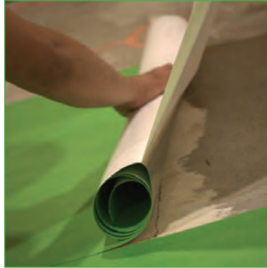
Remove Backing and GreenSkin™ Adheres Directly to Substrate
